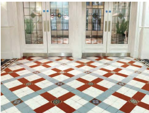
Aston Villa Football Club's Villa Park Stadium in Birmingham. The pattern in Red, Grey and White incorporating Liverpool is called Cliveden, was created especially for the location. Shown with Melville border ▲
